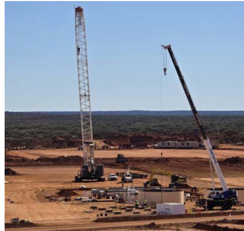
Figure 29: The 300t crane is built and ready to start construction of the plant. We can see ground being compacted in the background for the oxygen plant.
