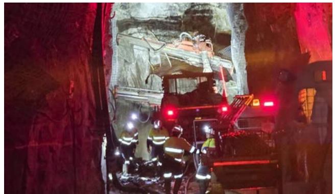
Figure 15: Jumbo at the decline face meshing. In some areas of the decline there is no stripping required.
