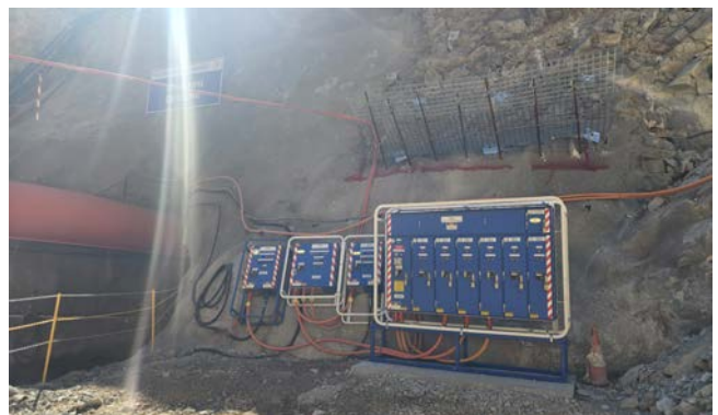
Figure 11: Surface infrastructure at the portal
