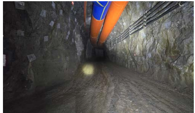
Figure 19: The access to the level. Nice and tidy, have a look at the ground conditions. This is what good looks like.
