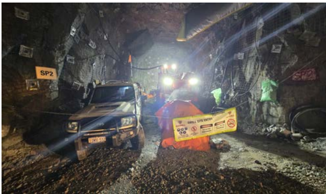
Figure 14: Underground rig is spinning.
