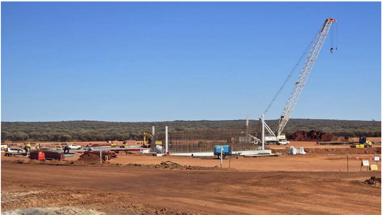
Figure 30: Fine ore bin formwork in the fore-ground with the 300t crane in the background.
