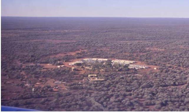
Figure 6: The camp build out is going well. Best in class mess facilities.
