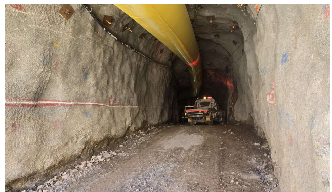
Figure 6: The United North Return Air-Way. Also picture perfect.
