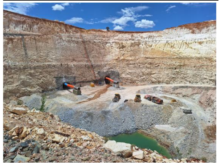
Figure 2: United North underground portals
