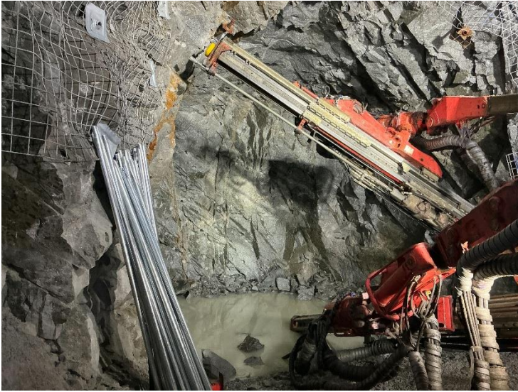
Figure 5: Jumbo bolting and messing development drive
