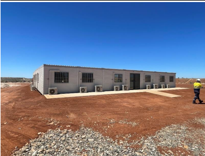
Figure 7: Underground mine offices
