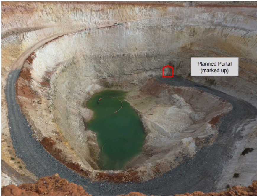
Figure 1: United North pit, road repaired, face meshed and Decline marked up
